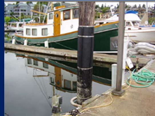
HDPE-wrapped treated wood pile
