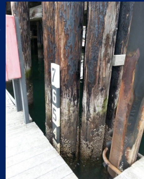
Creosote- treated piles
