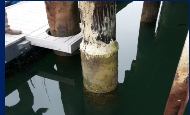
Pile repair using epoxy-filled fiberglass jacket
