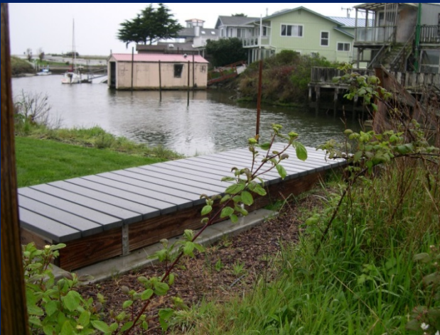
Composite decking on redwood framework
