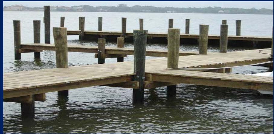
Treated wood decking, piles, & framework
